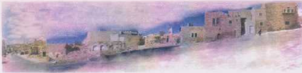
Panorama before intervention
