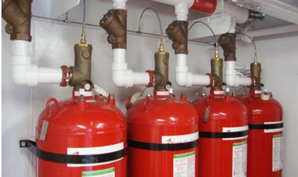
Figure (5.3) clean agent gases fire extinguisher.
