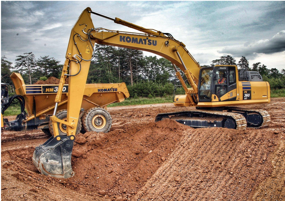
Figure 2. 1: An intelligent Excavator working in real workspace.
