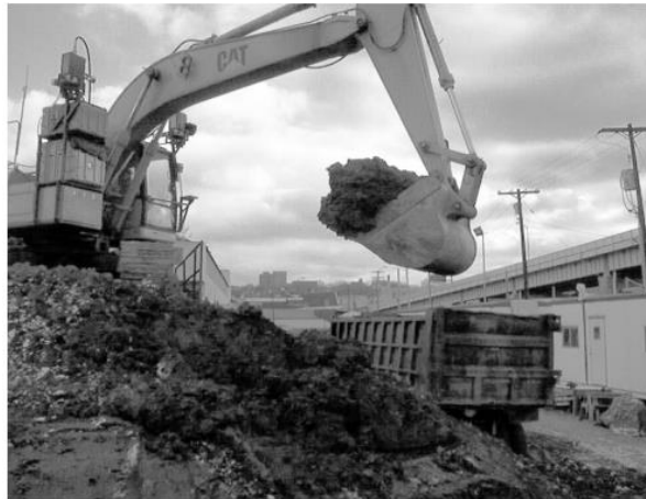
Figure 1. 1: Typical dig for truck loading.
