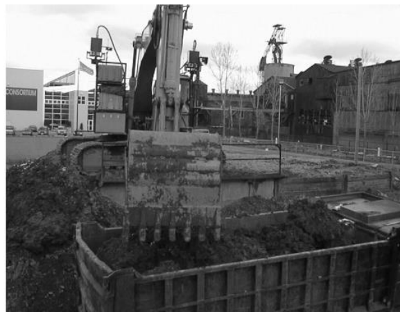
Figure 1. 2: Truck is loaded after six passes.
