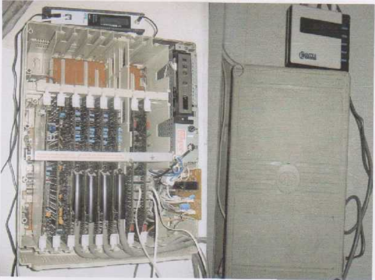
Fig. 5.2 Second Stage Testing
