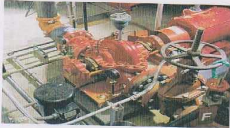
Figure (4.4): Horizontal split case pump
