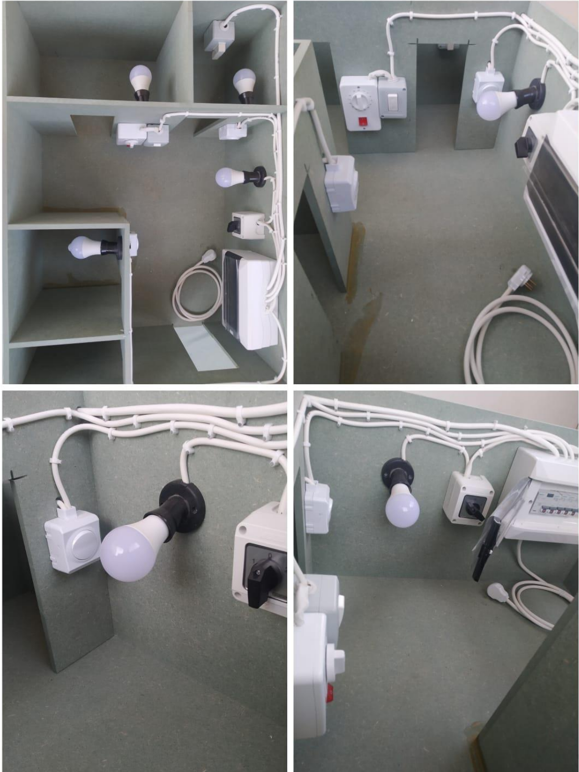
figure 5.1: The model simulates the fifth floor of the B-building in ppu with the application of the proposed system to it.
