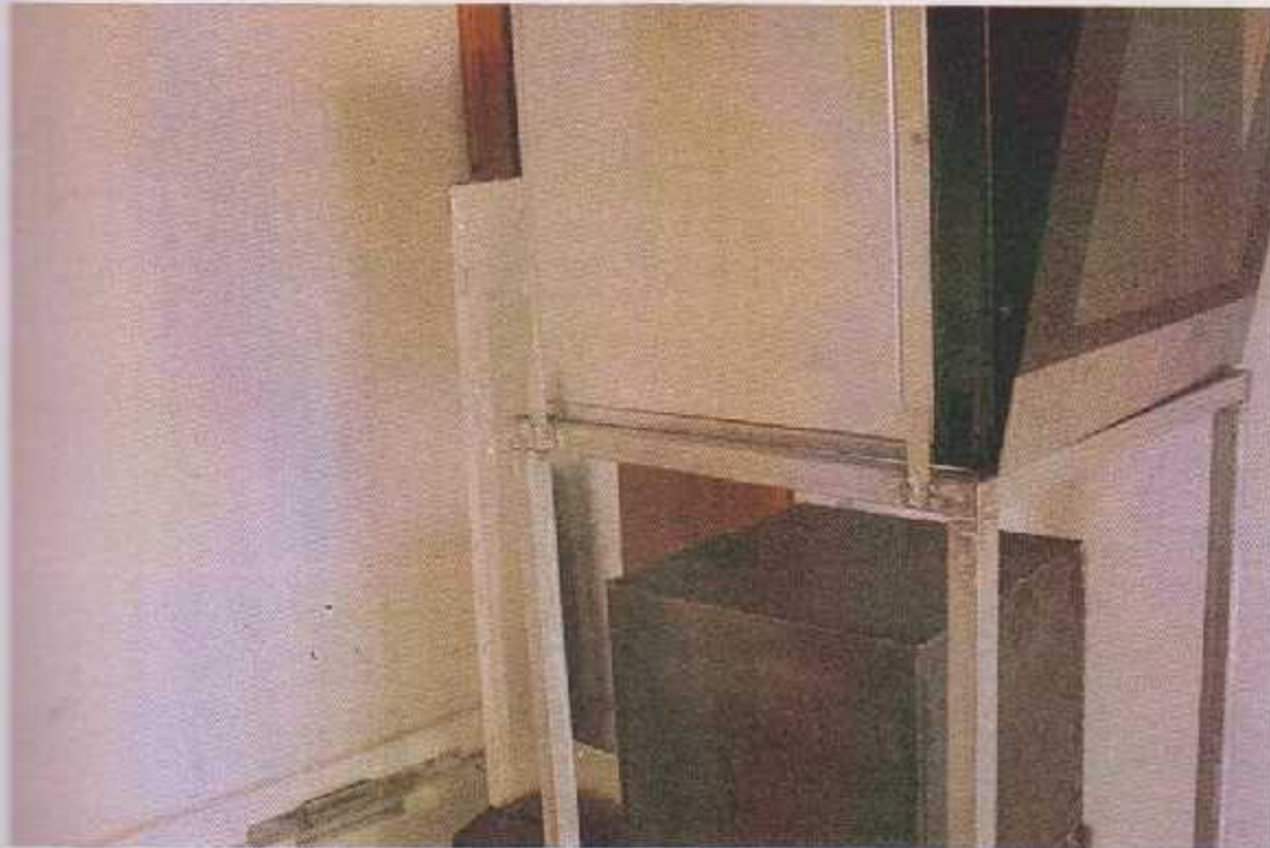
Figure 4.2: The whole system of cable insulators smelting furnace (another view).
