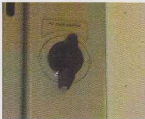
Figure 6-1 DC circuit breaker
