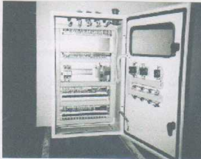
Figure 3.7: Typical PLC Control Panel
