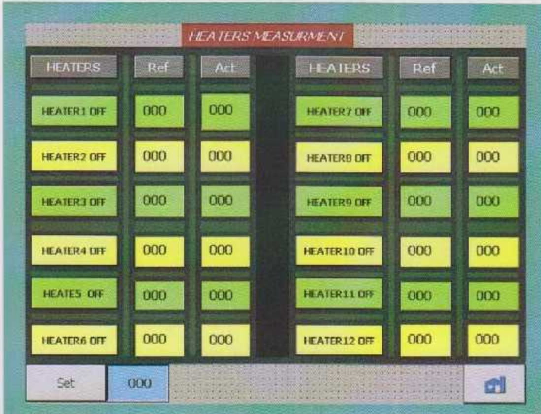
Figure (6.5): The heaters measurement screen.
