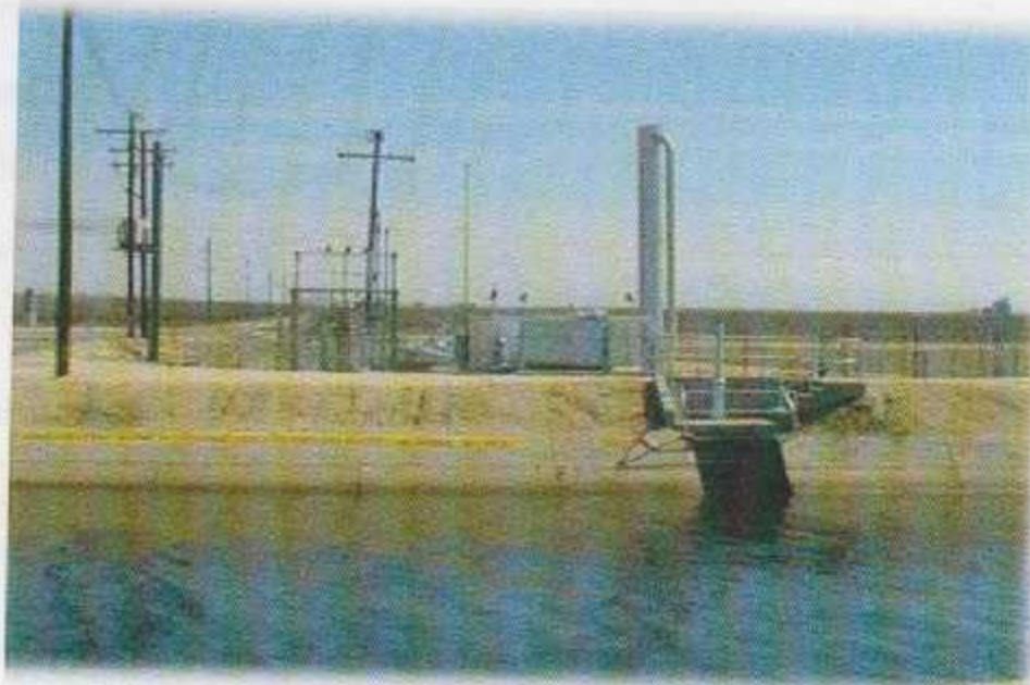
Figure 4.3: DFID turnout from the Friant Kern Canal that services an uphill section of the district.
