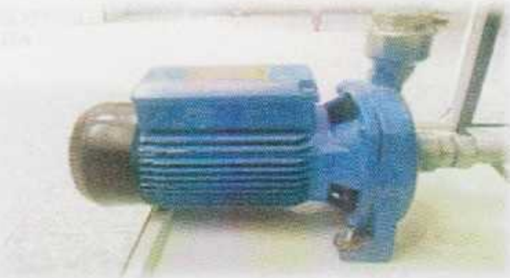
Figure 5.4: Three Phase Pump
