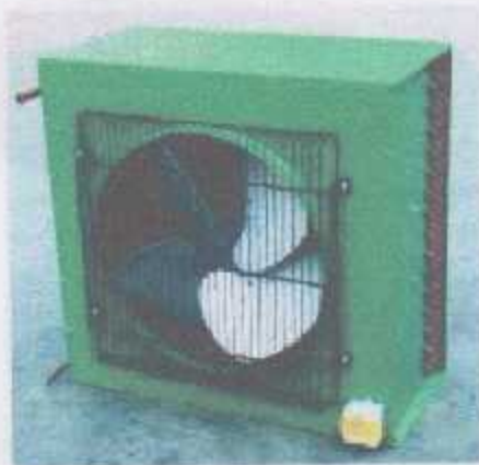
Fig (3.9) air cooled condenser
