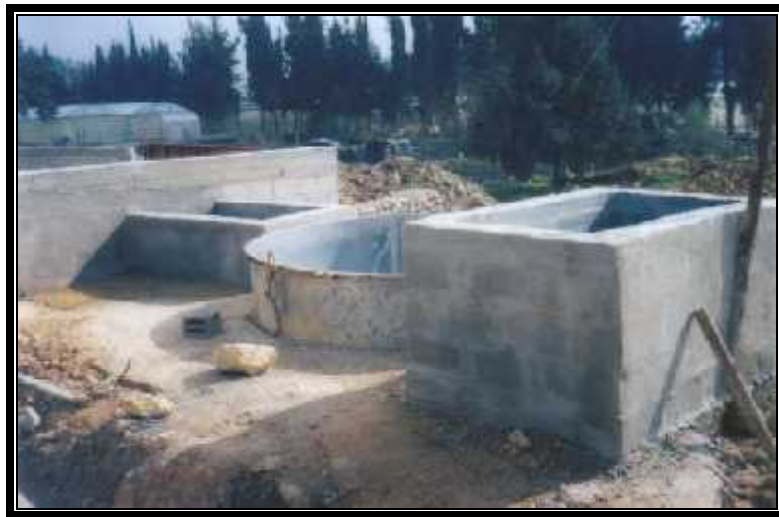
Figure A-11: Digester prior to floating dome installation
