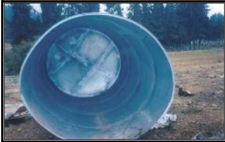
Figure A-13: Dome (inside view)
