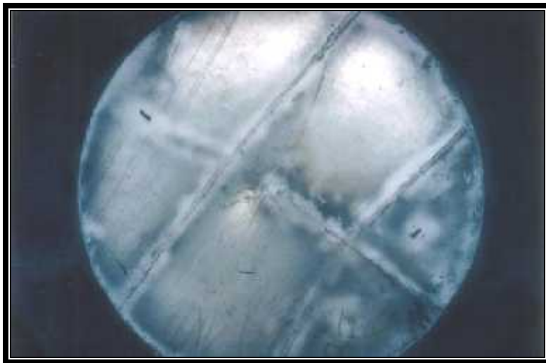
Figure A-8: Floating Drum ceiling from inside
