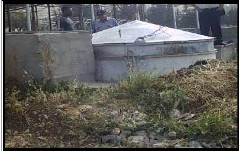
Figure A-16: 2 days installation of the plant
