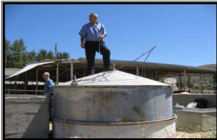
Figure A-17: AFC biogas plant (gas trapped in)
