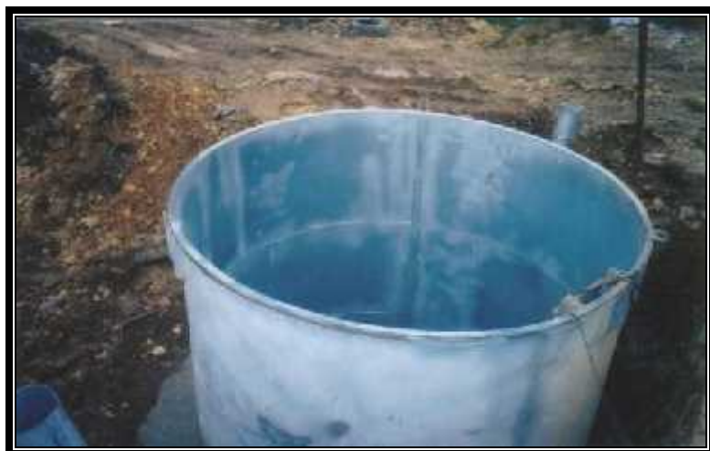
Figure A-15: Digester during installation
