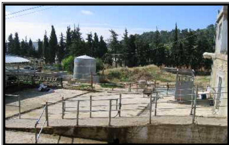
Figure A-18: General view of AFC plant
