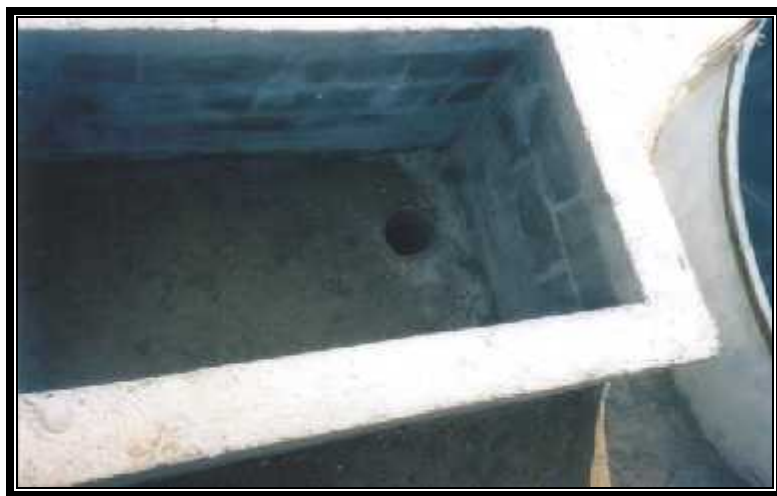
Figure A-9: Outlet pipe and 8" (with the floor level of the effluent receiving chamber)
