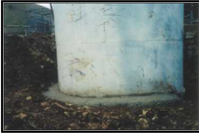
Figure A-7: Digester during installation in the pit.
