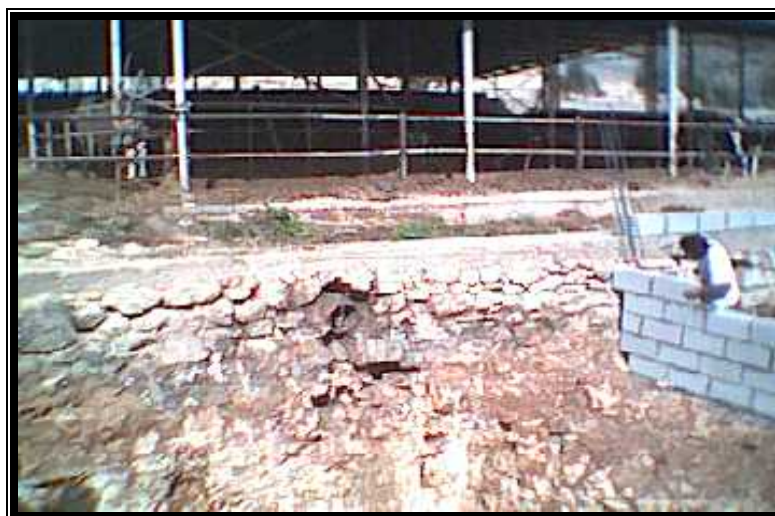
Figure A-3: The location of the pit near thr cow barn.
