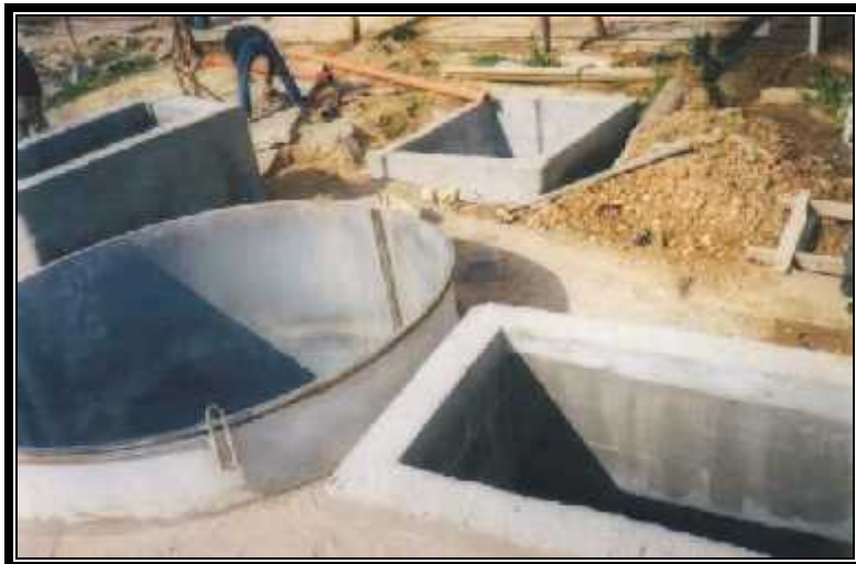
Figure A-14: Digester + the mixing chamber + outlet receiving chamber + barn flushing chamber (middle) does not connect to the digester.
