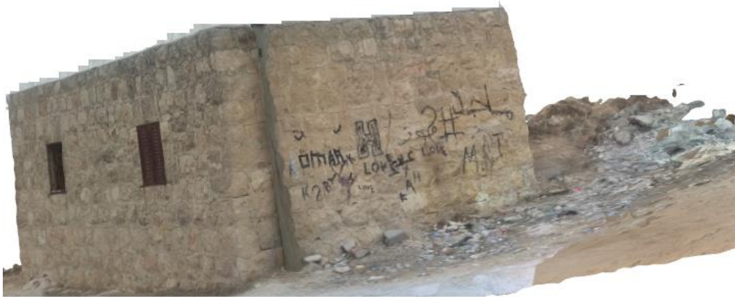
Figure(5.11) 3D model of the house by a variable distance from the house by Agisoft photo scan professional .
