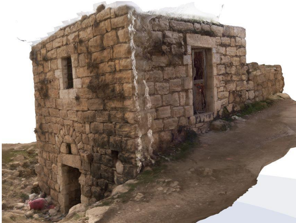
Figure(5.15) 3D model of the house by a variable distance from the house by Memento Autodesk software.
