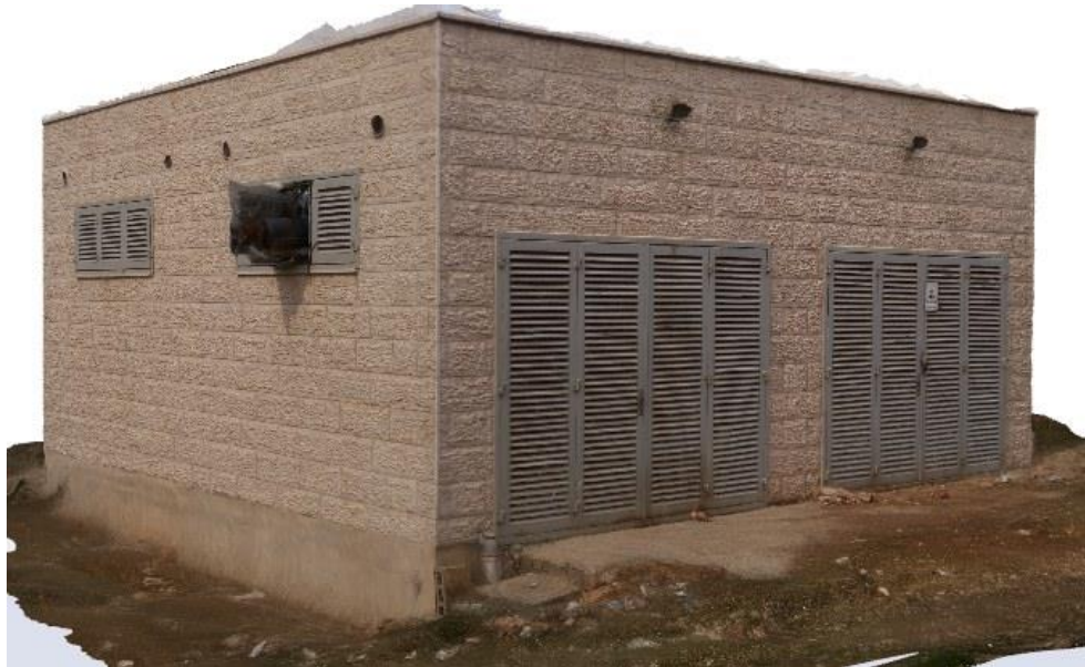
Figure(5.17) 3D model of motor room by a variable distance from the object by Memento Autodesk software.
