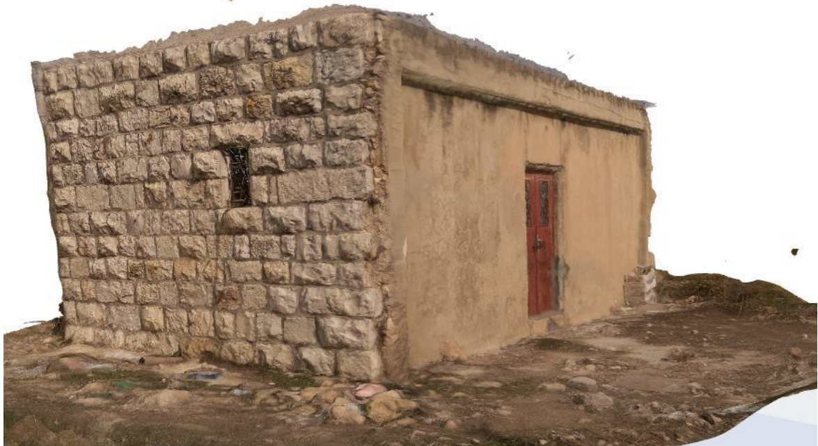
Figure(5.23) 3D model of the old house by a variable distance from the object by Memento Autodesk software
