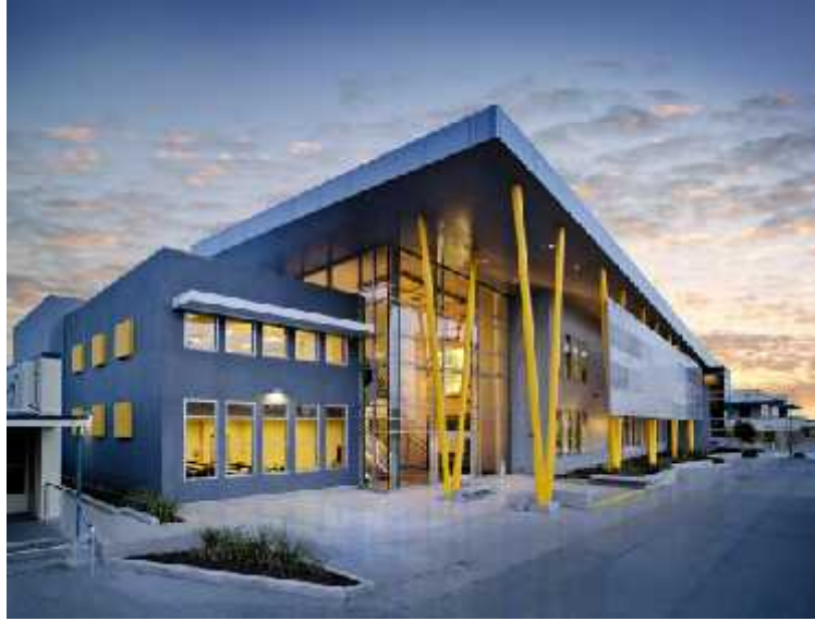
Edison Technical High School Academic Building ( - )
