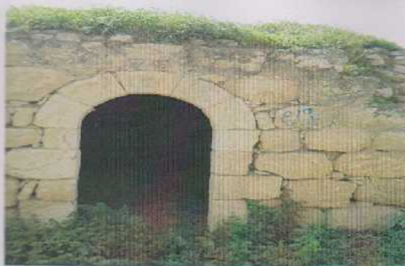
Figure (2.27): Building in moderate condition [ Project Team ].
