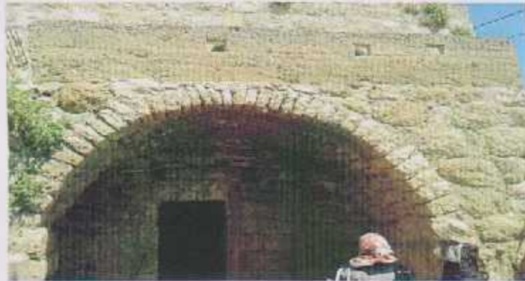
Figure (2.19): Abandoned old building [Project Team].
