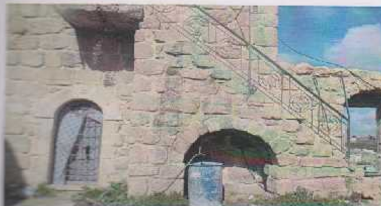
Figure (2.22): Three-story buildings [ Project Team ].
