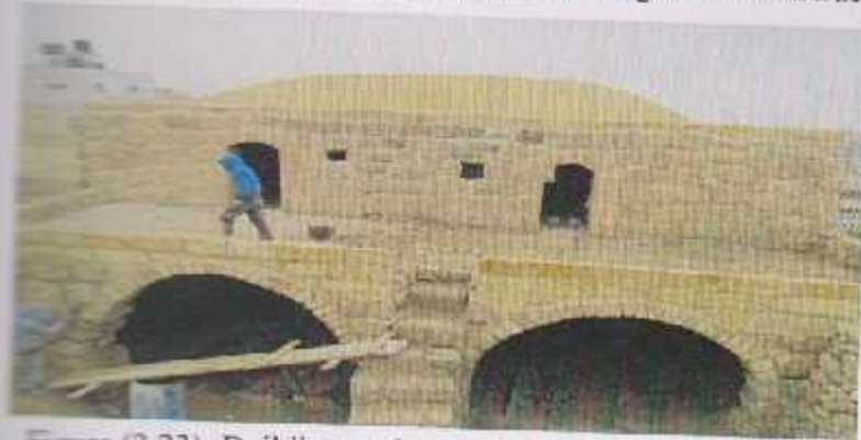
Figure (2.23): Building under construction [Project Team].
