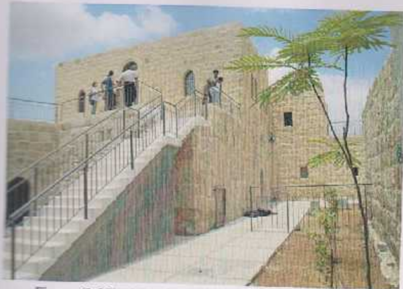
Figure (2.25): Completed building [ Project Team ].
