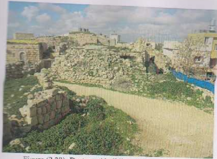
Figure (2.29): Destroyed buildings [ Project Team ].
