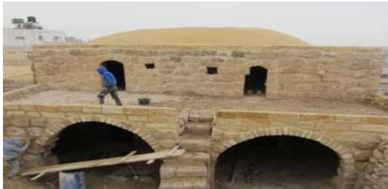
Figure (2.23): Building under construction [Project Team ].
