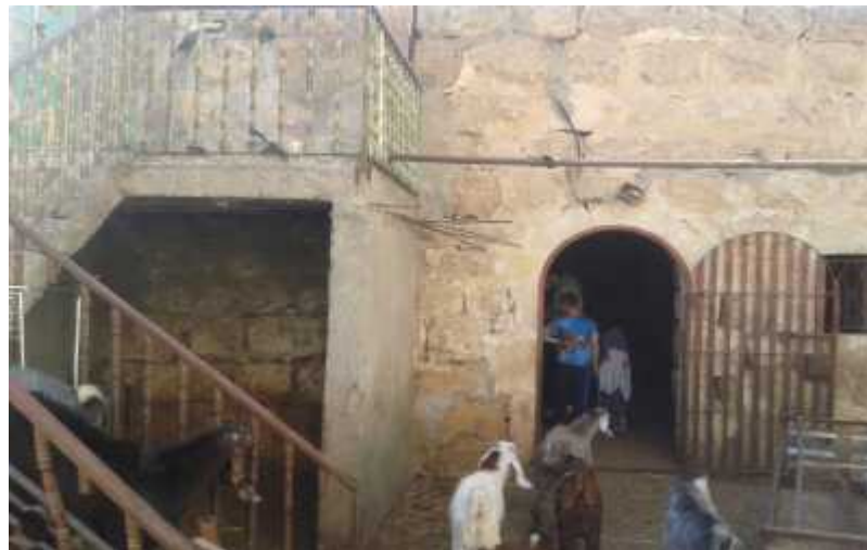
Figure (2.18): Old building for livestock breeding and animals[Project Team].
