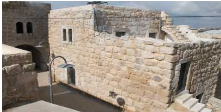
Figure (2.26): buildings in a good construction [ Project Team ].
