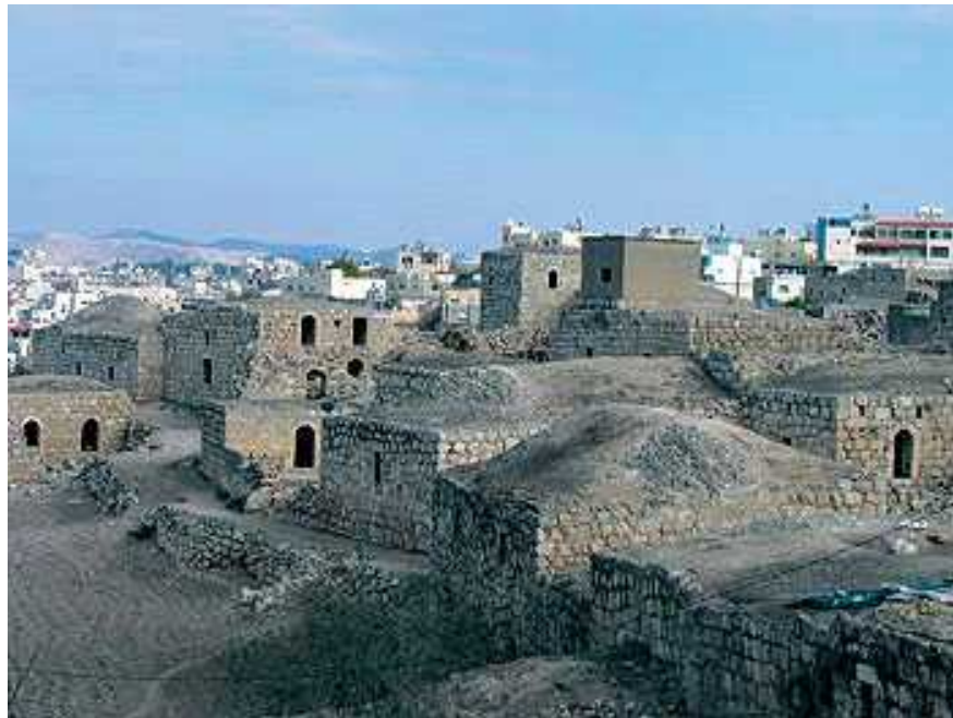
Figure (2. 1) General View of the of AL-Dahriya Old City[2].
