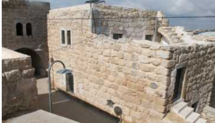
Figure (2.21): Two-story buildings [ Project Team ].
