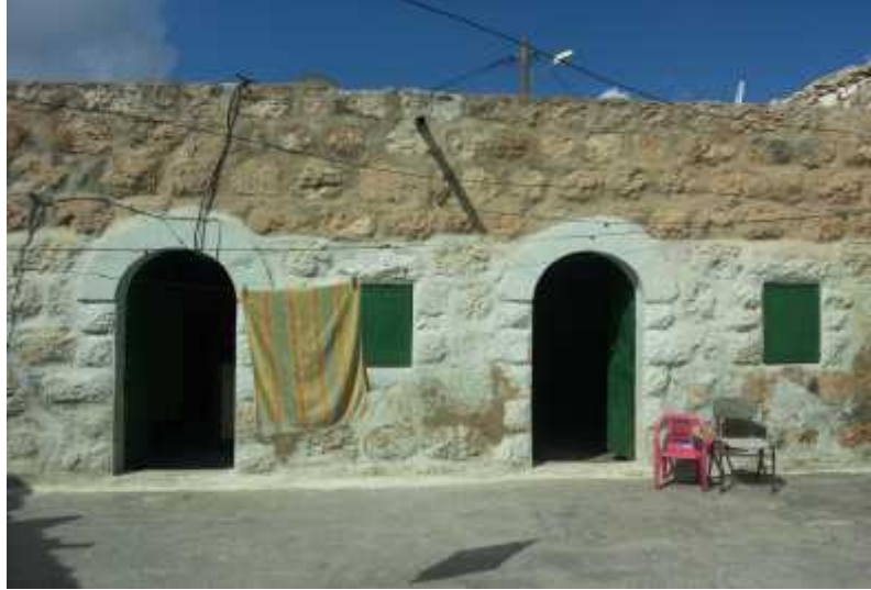
Figure (2.13): Old building for residential use [ Project Team ].
