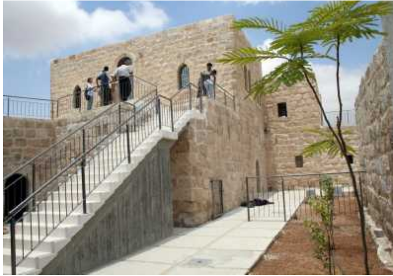
Figure (2.25): Completed building [ Project Team ].
