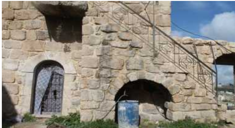
Figure (2.22): Three-story buildings [ Project Team].
