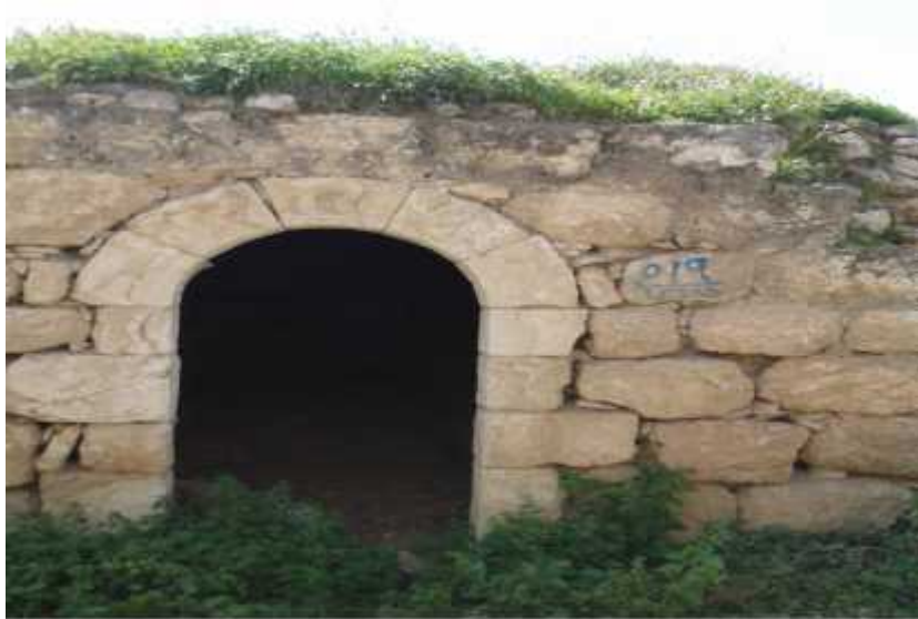
Figure (2.27): Building in moderate condition [ Project Team ].
