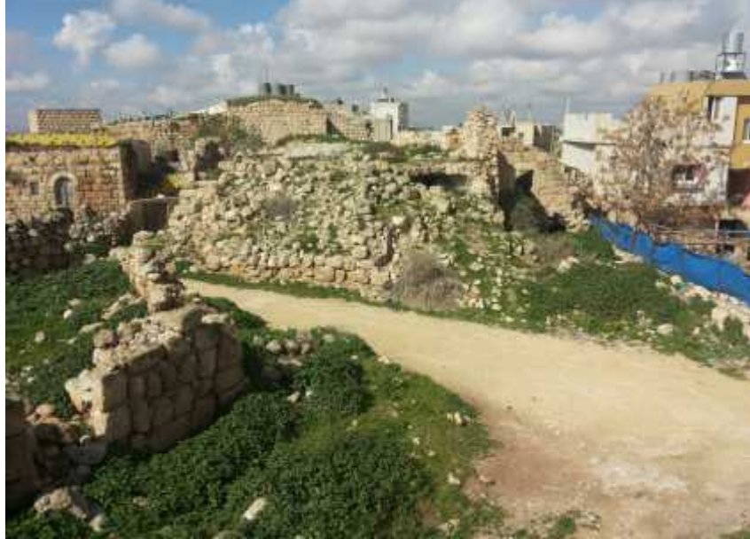
Figure (2.29): Destroyed buildings [ Project Team ].
