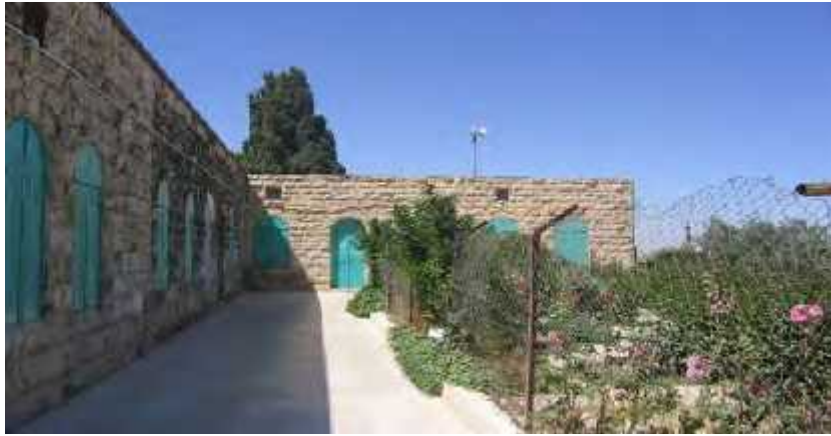
Figure (2.15): Old building for educational use (Al-Dahriya School)[ Project Team ].
