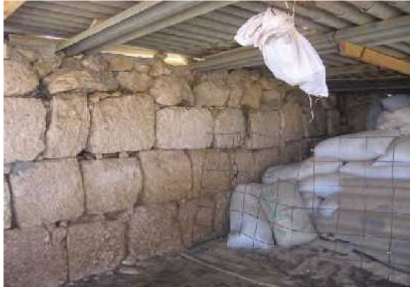
Figure (2.17): Old building for storing [Project Team].
