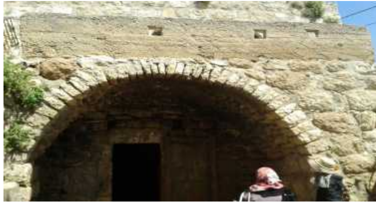
Figure (2.19): Abandoned old building [Project Team ].
