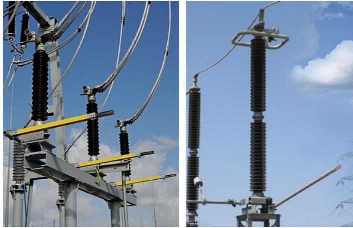
Figure 3.10: Earthing switches type TEC and TEB
