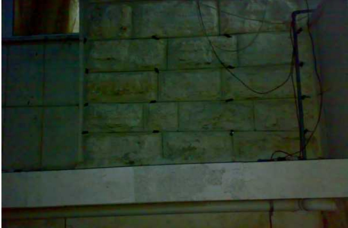
Figure 4.35: Outer wall in Class twelve
