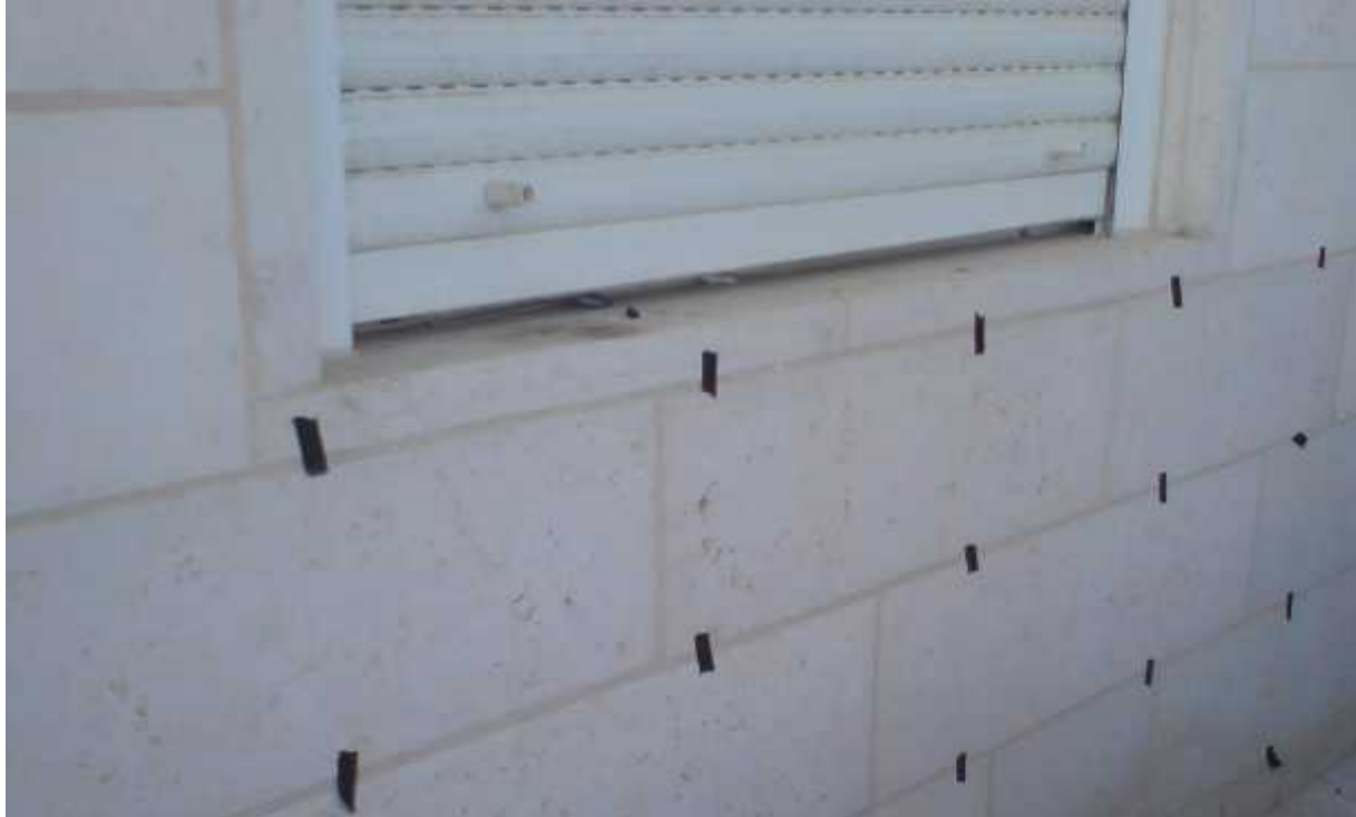
Figure 4.29: Outer wall in Class ten
