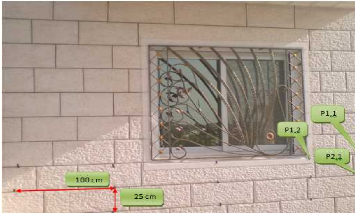
Figure 4.23: Outer wall in Class eight
