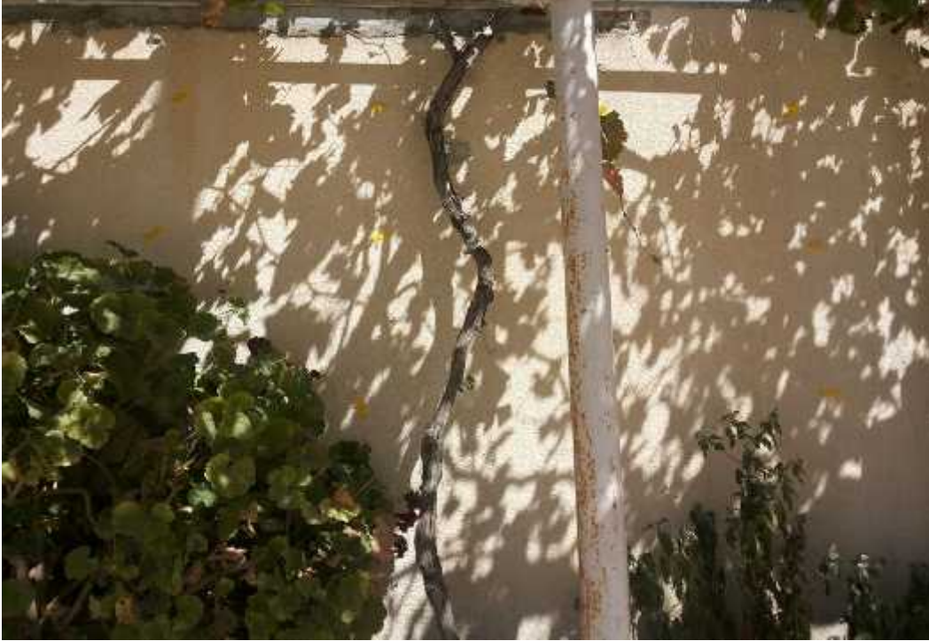
Figure 4.2: Outer wall in Class one
