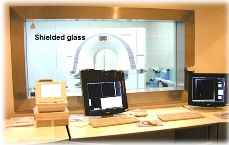
Figure 3.23: The Operator's Room Glass [45]
