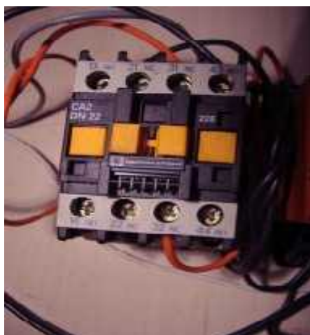
Figure (4.1): Contactor
