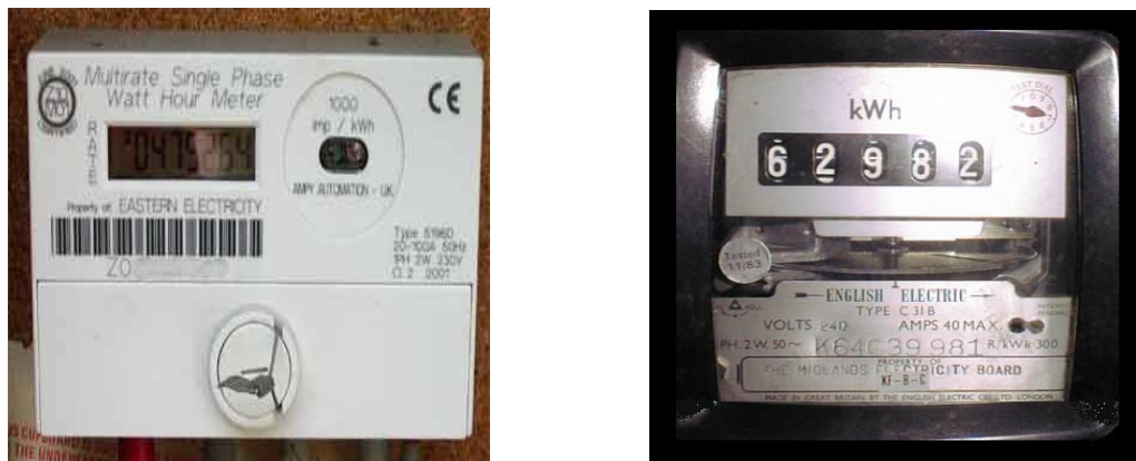
Figure 2.1: Different kinds of electricity meters.
