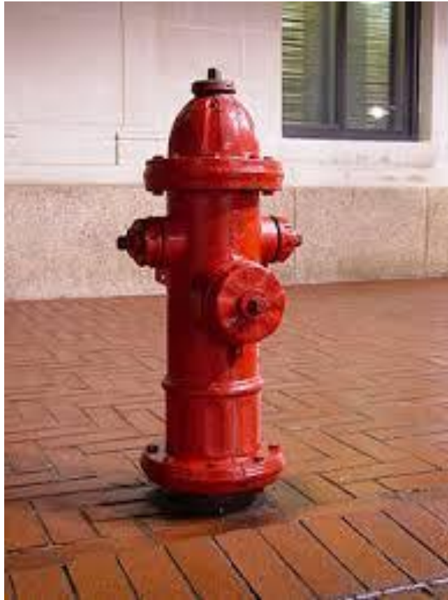
Figure (6.4) Fire Hydrant
