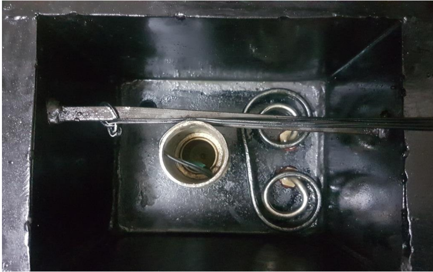
Figure 7.2 cleaning the tube.
