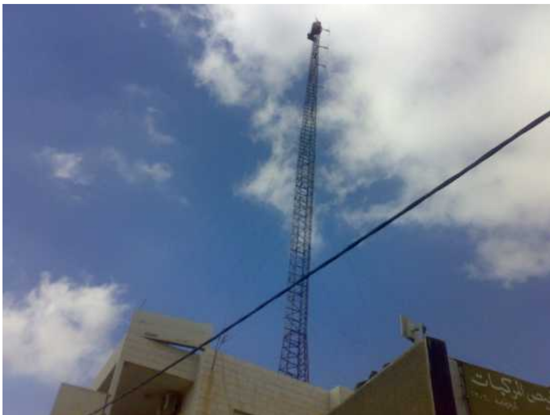
Figure.4.27: Alhoria FM radio station.
