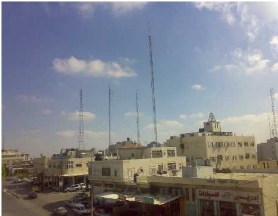
Figure 4.22: Broadcasting towers view at N 31°33'26.41"; E 35° 5'43.41".
