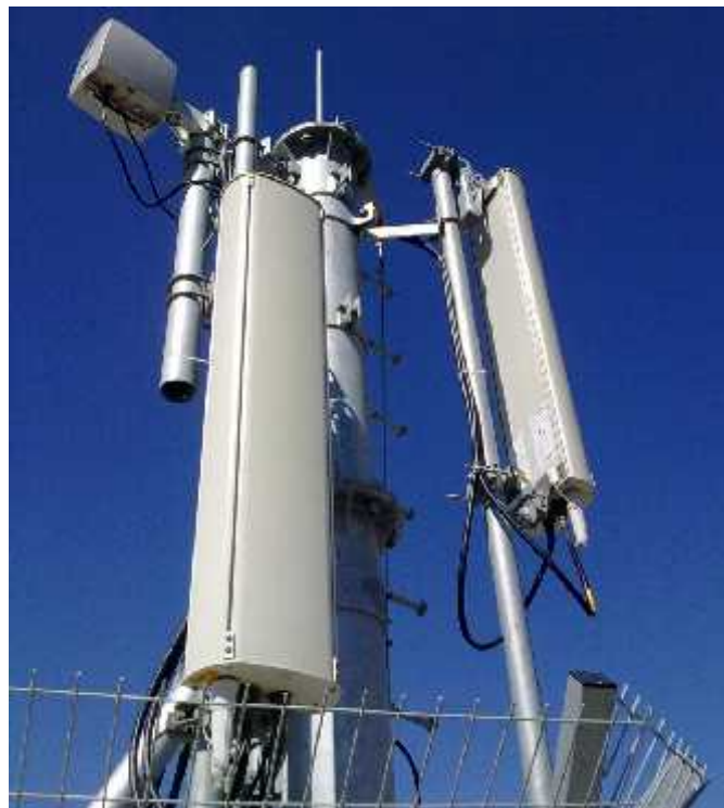
Figure 4.16: JAWWAL outdoor macro cell antenna.
