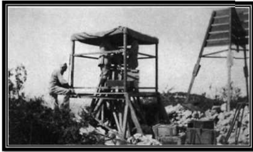
Figure (2-5): Survey post on Jebel Jarmaq (Mount Meron) for the geodetic junction between Palestine and Syria and Lebanon {1}.
