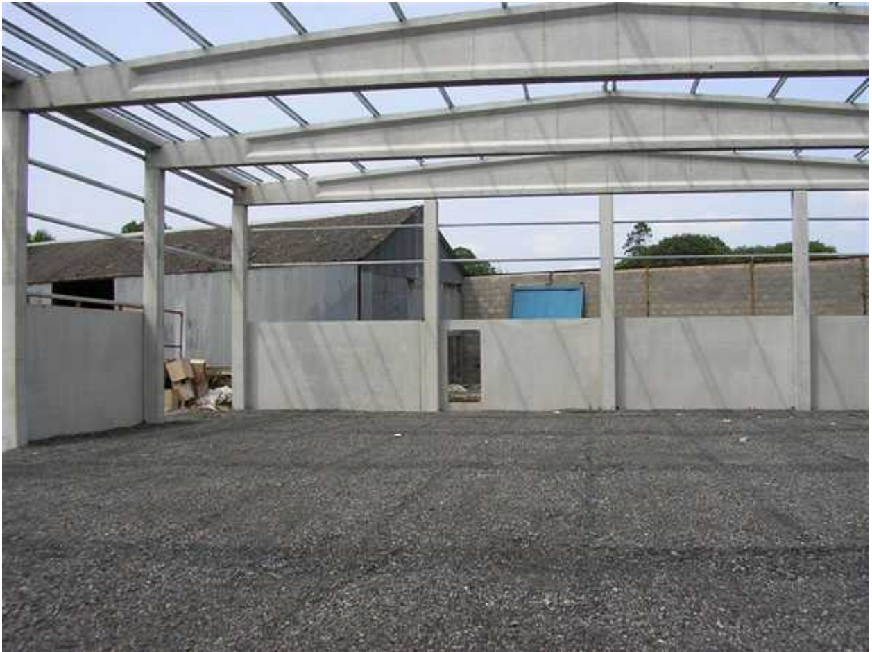
Figure (3-13): Frame Structure.
