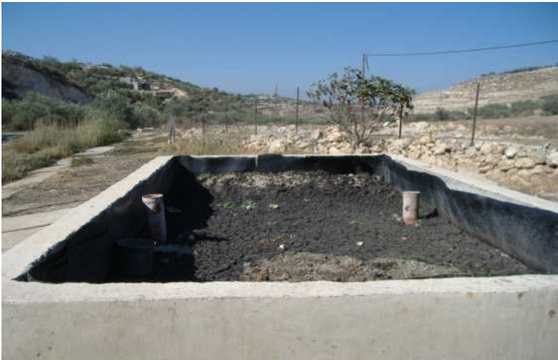
Fig (4.10): Sludge Drying Bed at Kharas Wastewater Treatment Plant
