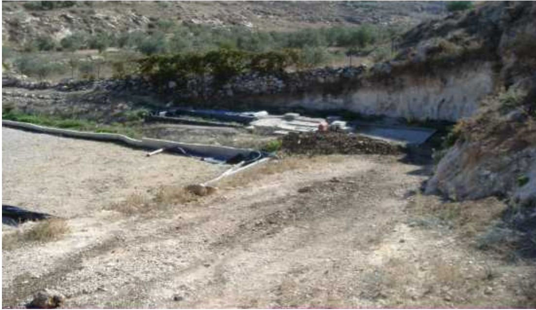
Fig (B.17): Wastewater Treatment Plant at Nuba Village
