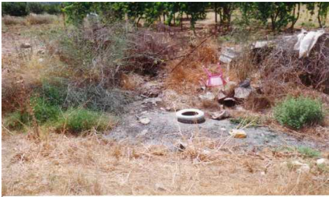
Fig (4.12): The Situation Before the Plant Construction
