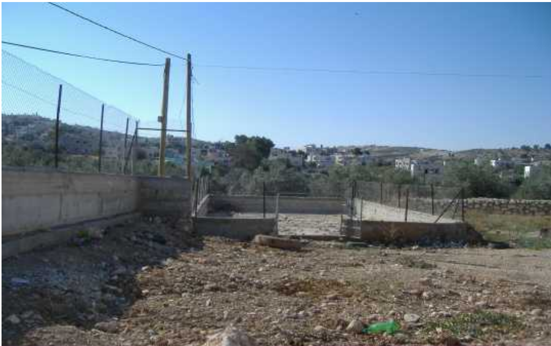
Fig (B.10): Wastewater Treatment Plant at Deir-Samit
