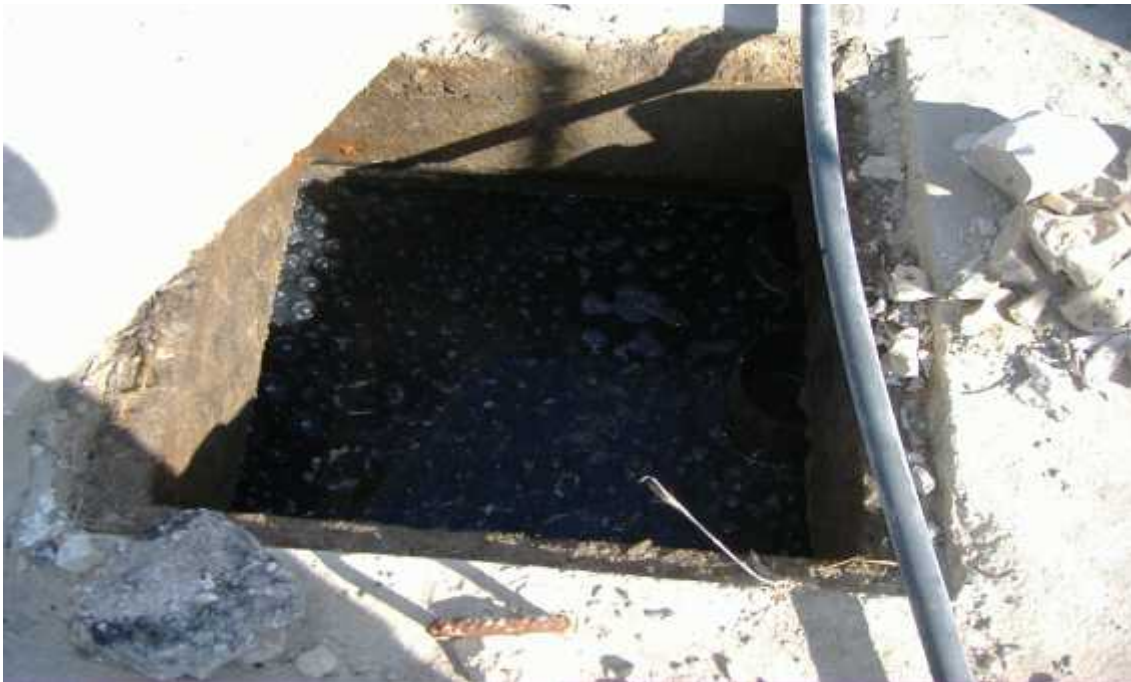
Fig (B.12): Anaerobic Septic Tank
