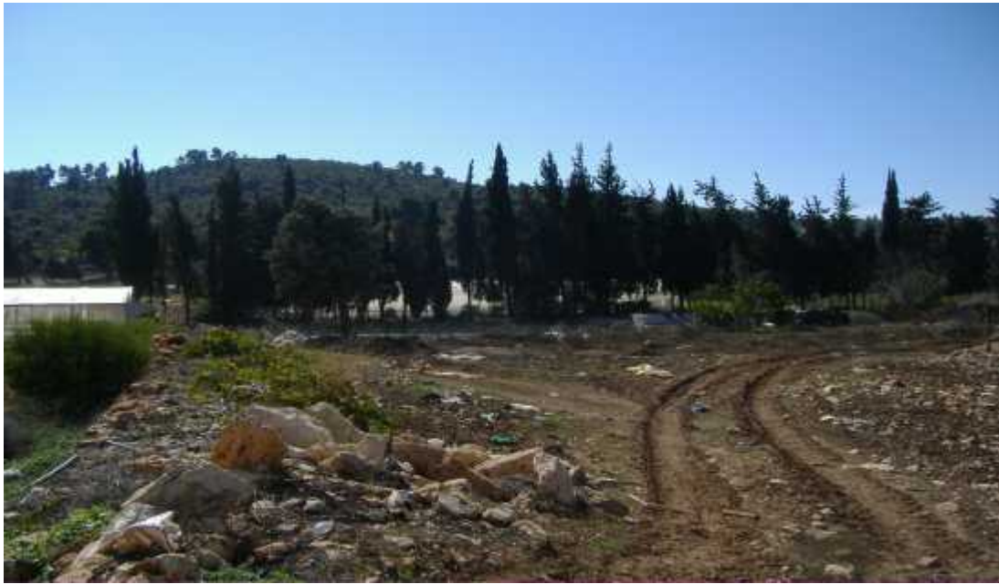
Fig (B.25): Al-Aroub Wastewater Treatment Plant
