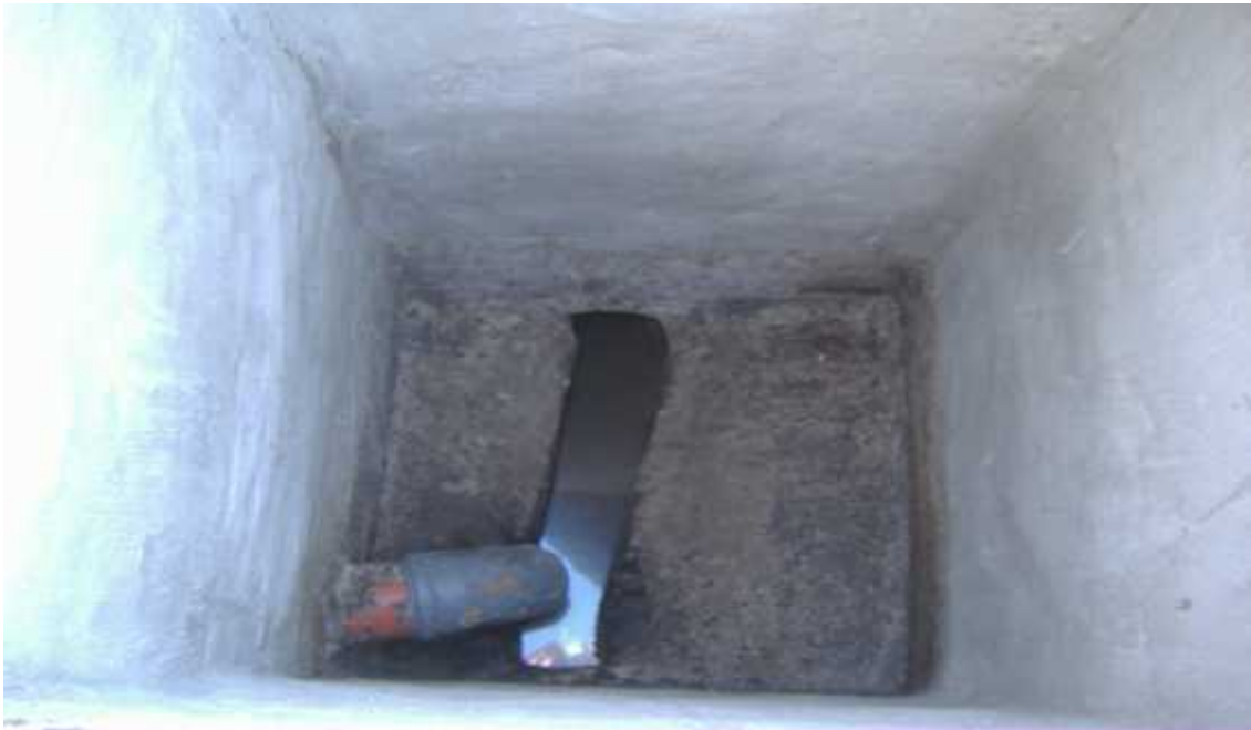
Fig (B.16): Storage Tank
