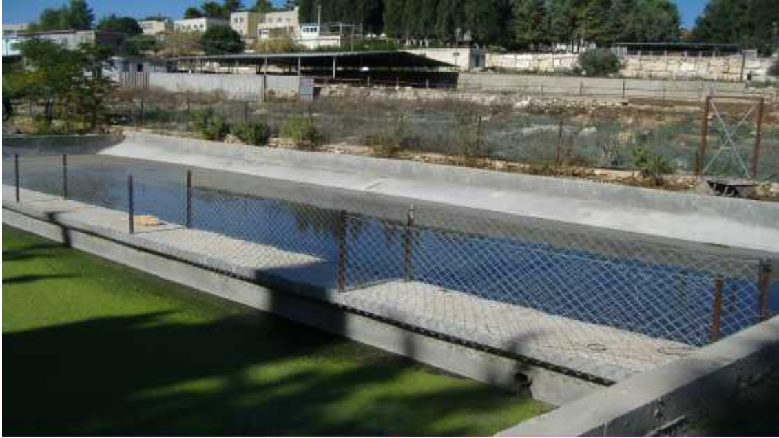
Fig (B.27): Treatment Process by Duckweed Ponds
