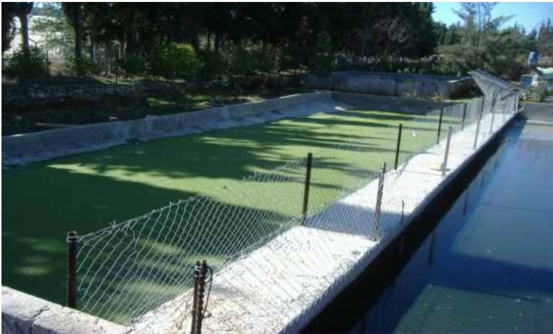
Fig (B.28): Duckweed Ponds at Al Aroub WWTP
