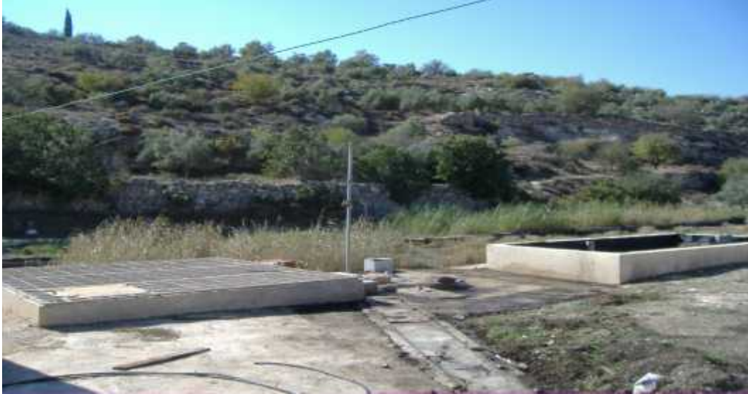
Fig (B.1): Wastewater Treatment Plant in Kharas Village
