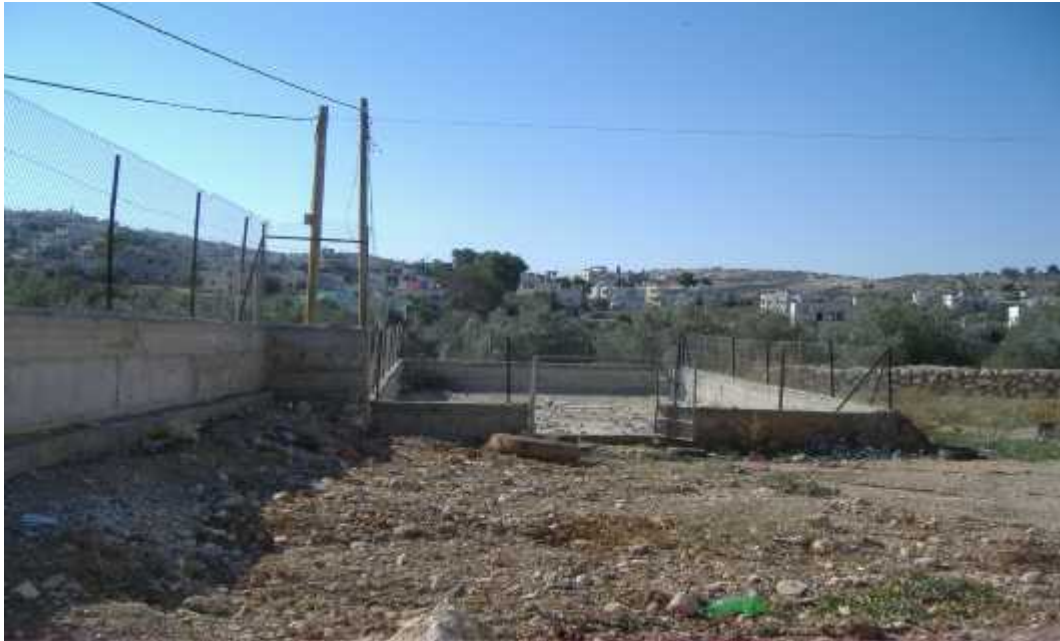
Fig (4.13): The Site of Wastewater Treatment Plant in Deir Samit Village
