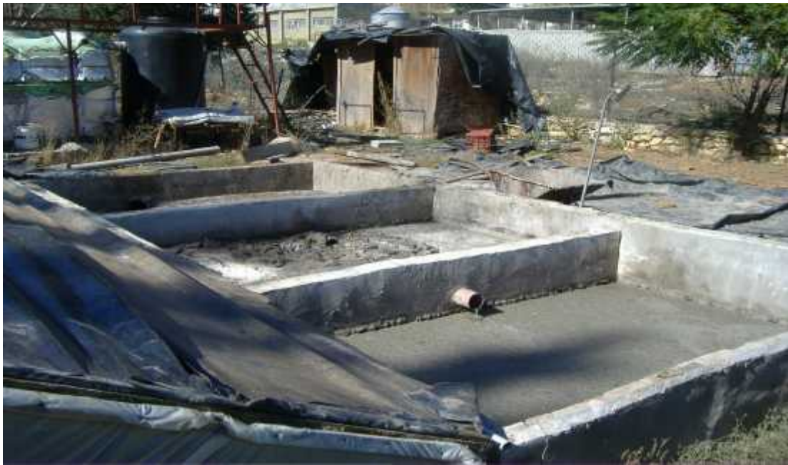
Fig (B.26): Settling Tanks at Al Aroub WWTP
