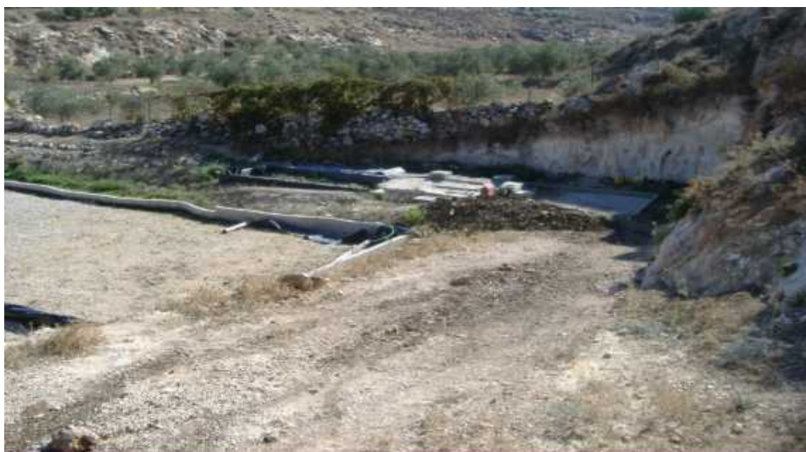
Fig. (4.20): Wastewater Treatment Plant in Nuba Village
