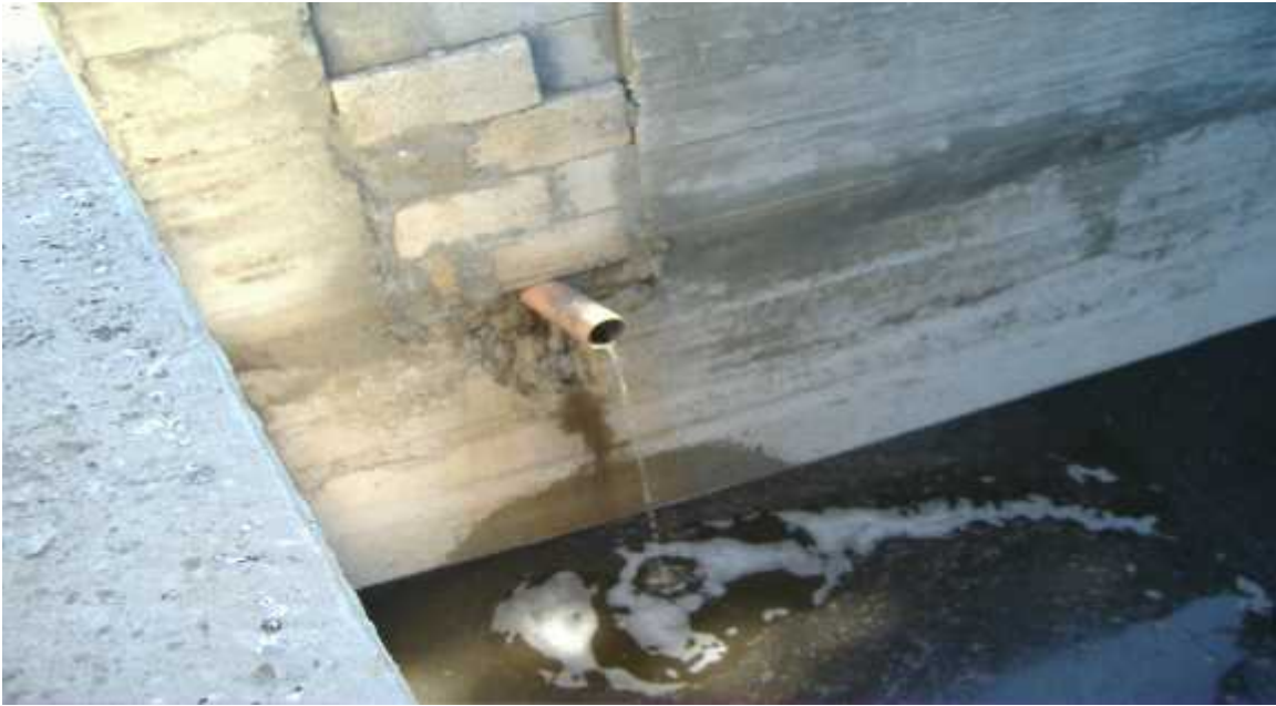
Fig (4.35): Storage Tank at Al Aroub Treatment Plant
