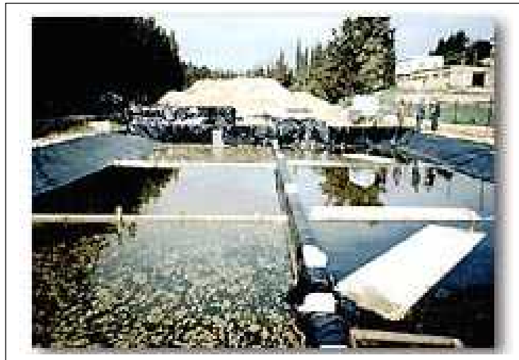
Fig (4.28): Al-Aroub Wastewater Treatment Facilities, (MOFAJ, 1999)
