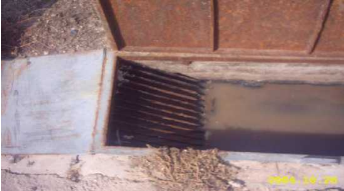
Fig (4.3): Picture of Bar Screen and Channel
