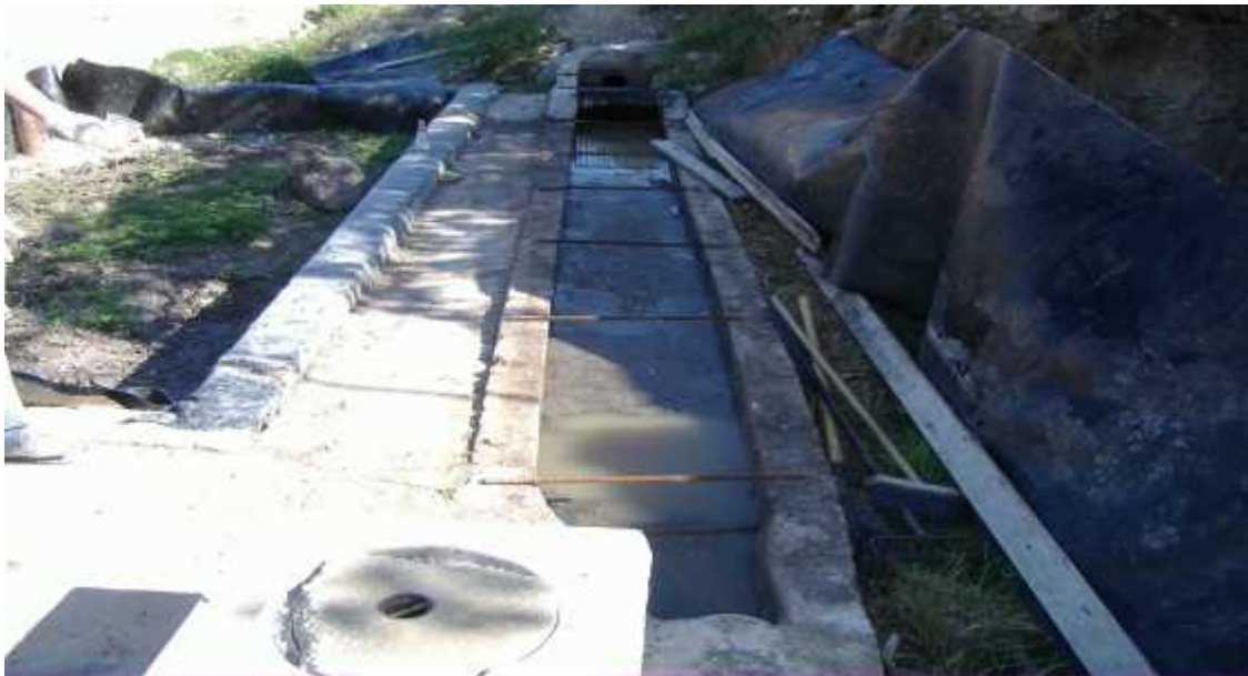
Fig (4.22): Picture of Screening and the Channel
