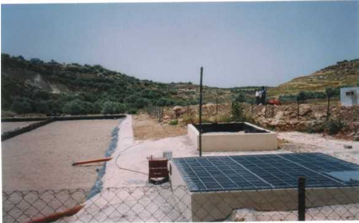
Fig (4.2): General View of the Wastewater Treatment Plant in Kharas Town
