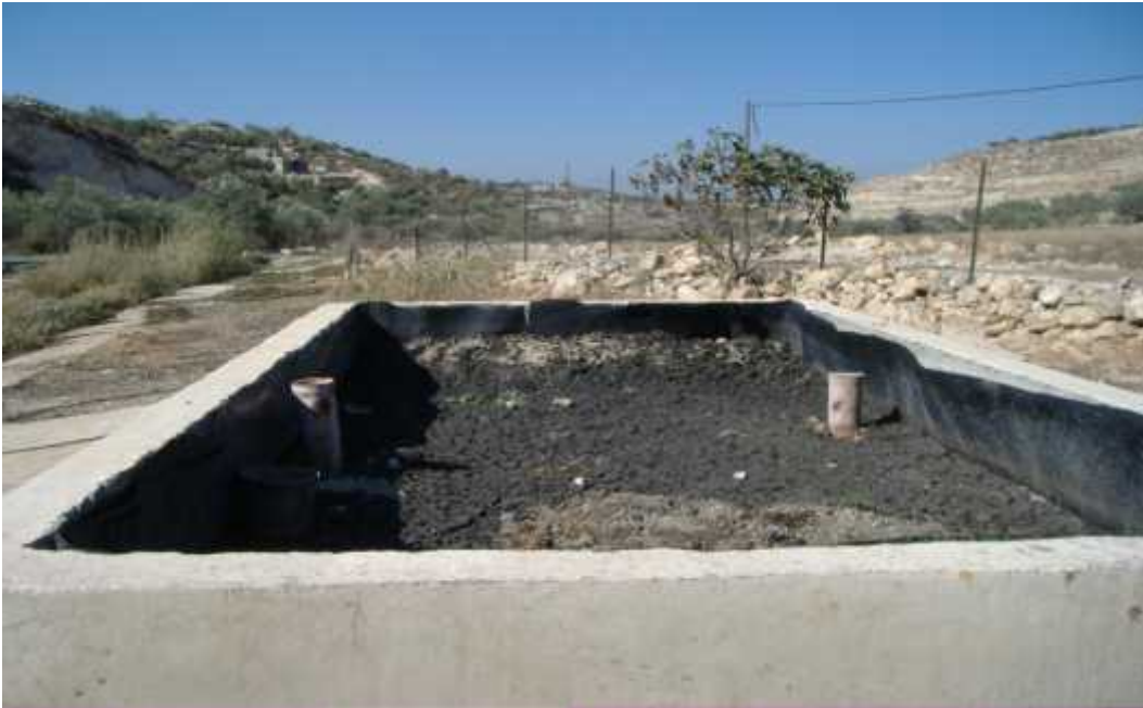
Fig (B.4): Sludge Drying Bed at Kharas WWTP
