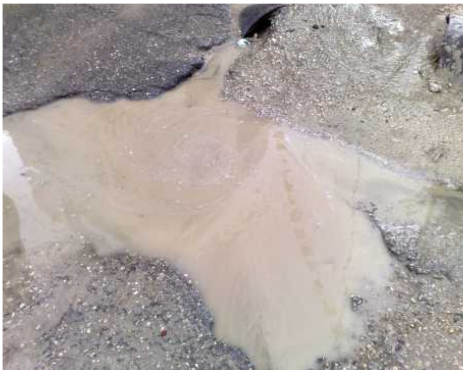
(Figure 3.6) Accumulative of Water at culvert.
