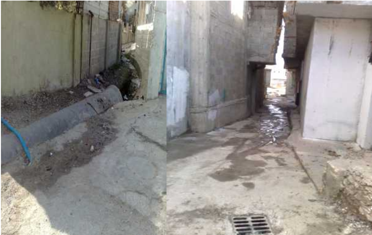
(Figure 3.5) A Culvert crossing the camp in left image, and the way where it cross "beside the wastewater" in right image
