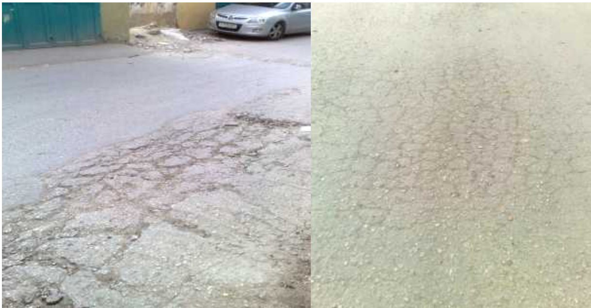
(Figure 3.7) Improper of road slopes, and asphalt cracks
