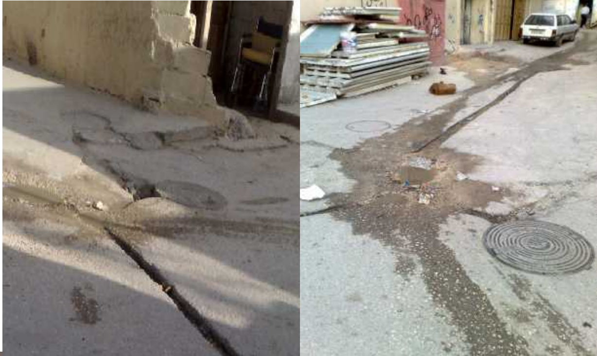
(Figure 3.4) Infiltration of rainfall to wastewater network.
