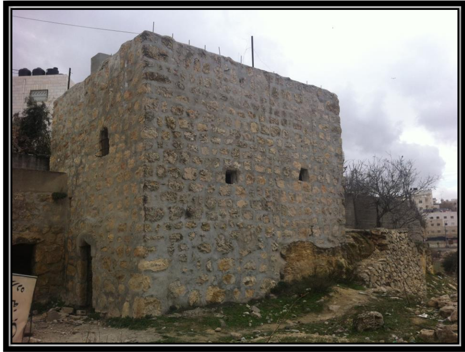
Figure (6 - 30) Old building
