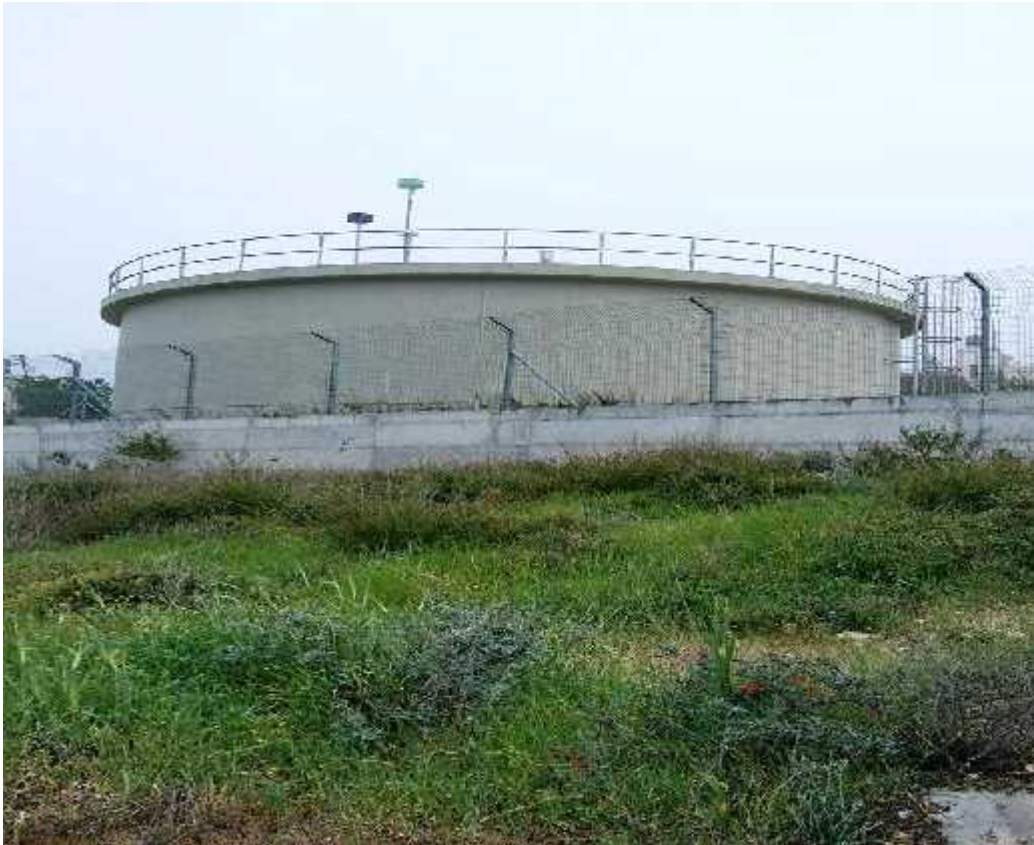
figure (3.7): pictures of Sourif tank
