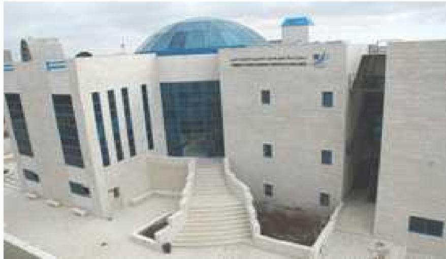
Figure (1.2) a photo of the glass dome of the building
