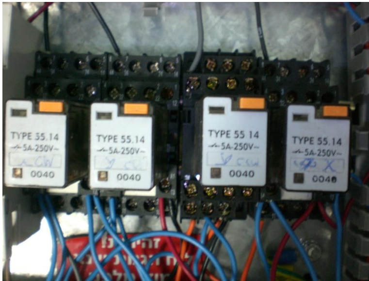
Figure 4.5 Relay for the System
