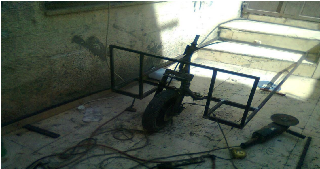
(a) Installing of steering system.
