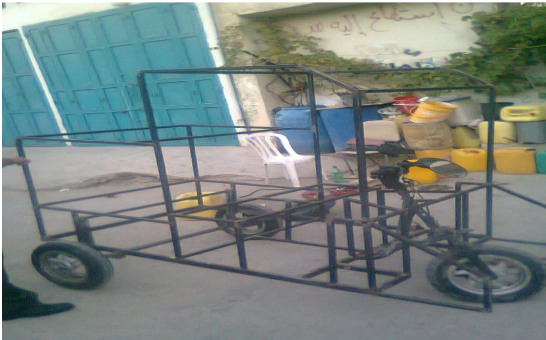
(d) Another view of chassis with complete installed rear axle and steering system.
