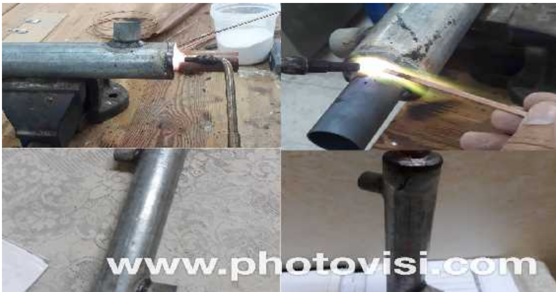
Figure 3.5: Pipe welding with each other .
