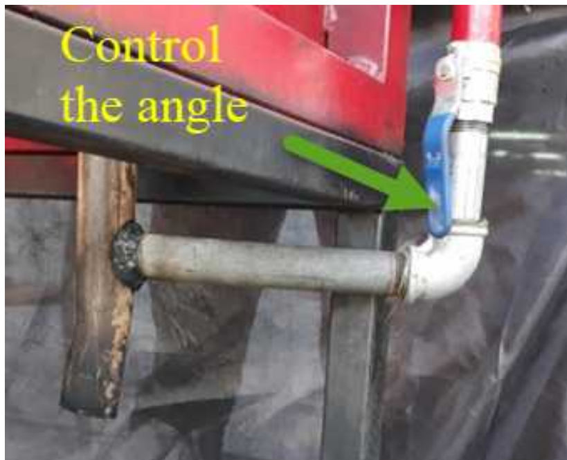
Figure 5-2 recycled exhaust gases mass flow with different angle We have compensated the denominator Air mass flow in the equation below to calculate velocity of airflow
