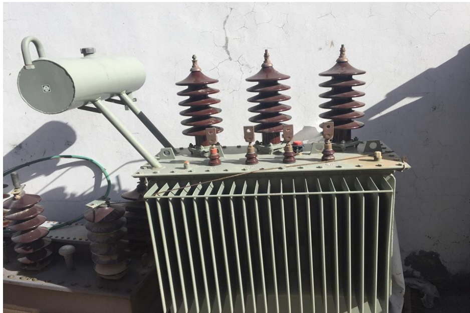
Figure2.6: Three-phase transformer
