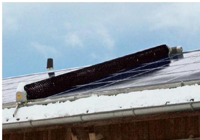
Figure 2-6: Sun Brush full automatic cleaning over solar panels
