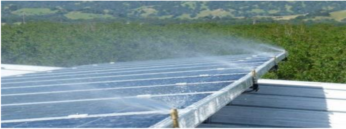
Figure 2-2: Heliotex cleaning technology using water and soap to clean the surface of PV panels
