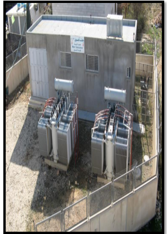
Figure (2.12) :(a) Switchgear in West (S/S) (b):Power Transformer in West (S/S)
