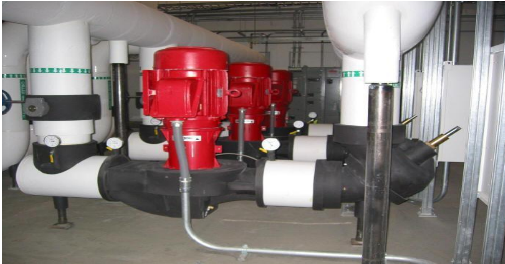
Figure 5.6: Inline fire pump
