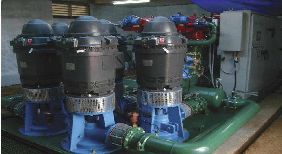
Figure 5.8: Vertical turbine pump
