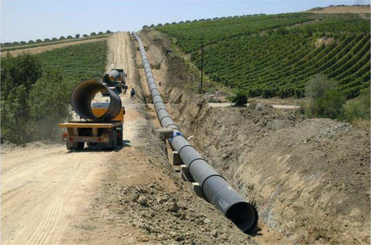
Figure 4. 2: Sub-project in Taksbt in Algeria
