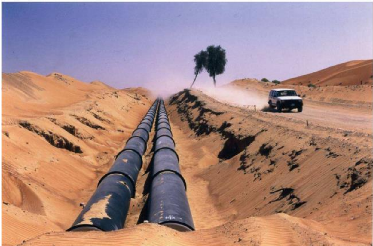
Figure 4. 1: Sub-project Classic Pipes in Taweelah in the UAE
