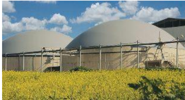
Figure (3.2): Biogas plant.
