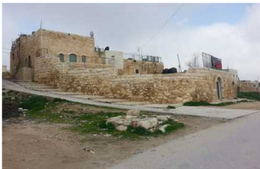
Figure 4.15: building in good construction
