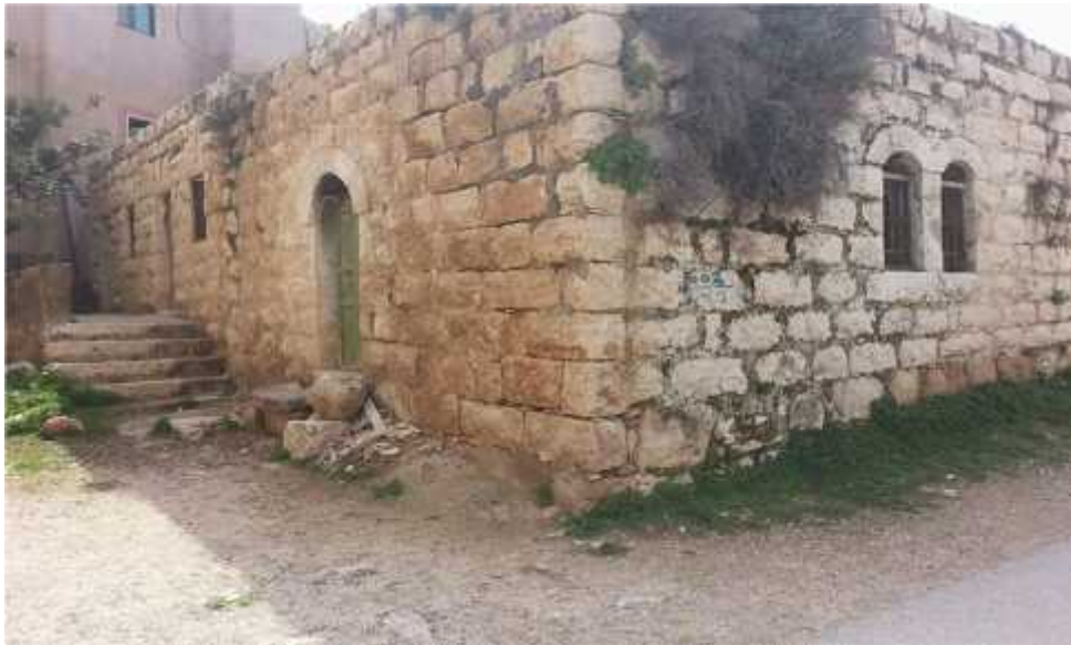
Figure 4.16 : building in moderate condition.
