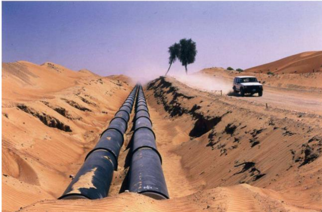
Figure 5. 1: Sub-project Classic Pipes in Taweelah in the UAE
