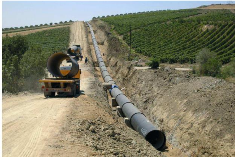
Figure 5. 2: Sub-project in Taksbt in Algeria
