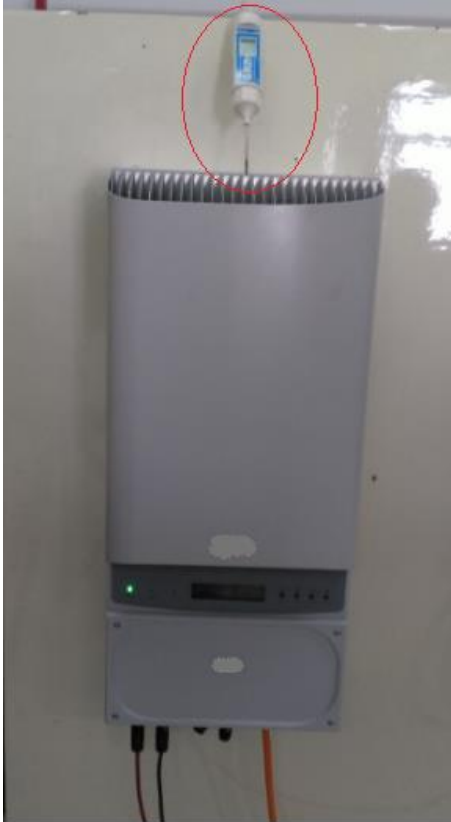
Fig 4.2: Thermometer with European Inverter.
