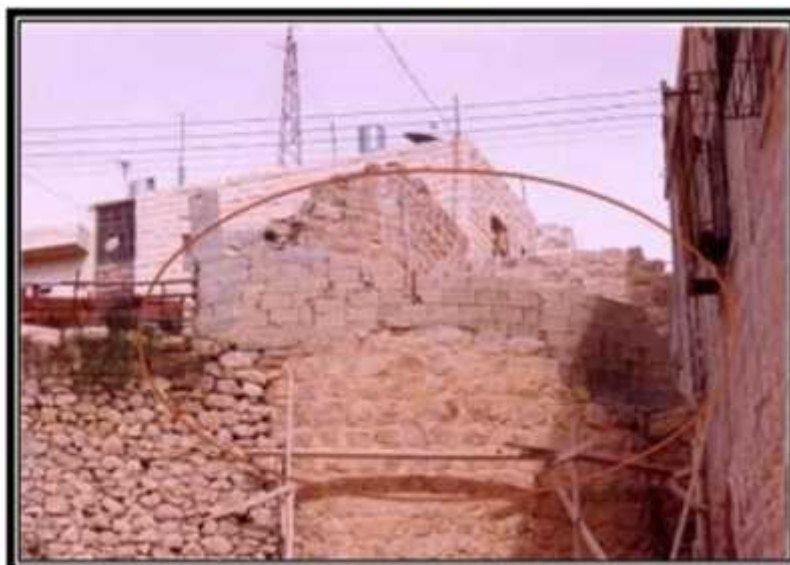
Figur 7 : shows the cement brick which is inconvenient for it's surrounding (the old original stone )
