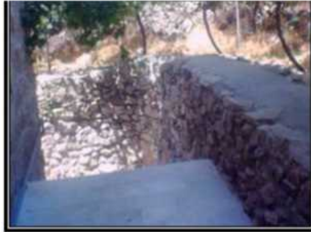
Figur 8 : shows the corridors after the renovation .
