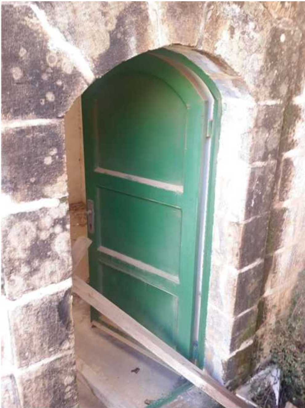
figure 7.3: We will renovate those walls after cleaning the stone and using the suitable material of mortar and preparing the doors and windows . Source : by the researcher .
