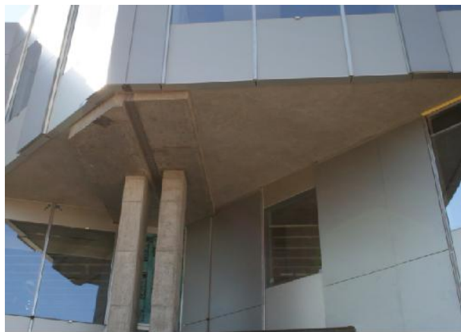
Figure (3.13): Expansion joint
