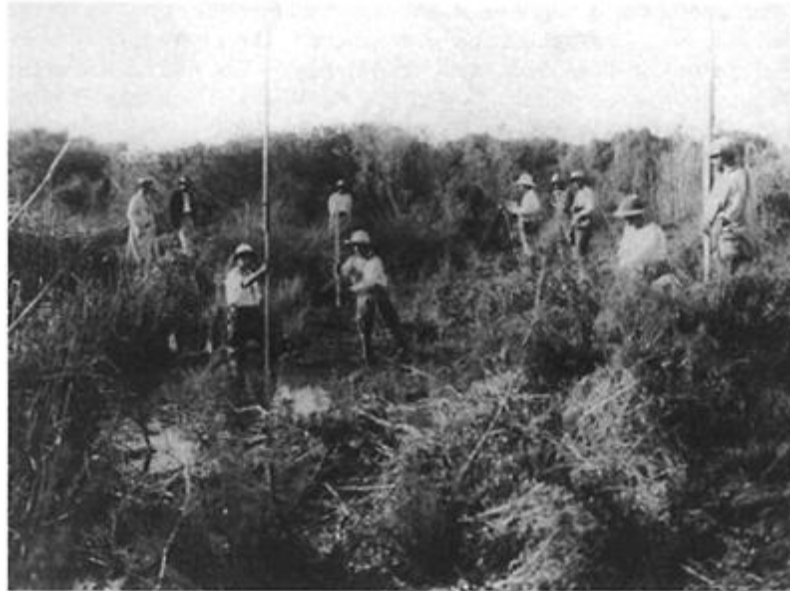
Figure (2.7): Leveling survey [4]
