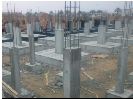
Figure(3- 7): Isolated Footing
