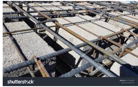
Figure(3- 4):Two way ribbed slab
