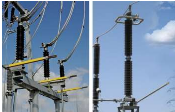
Figure 2.12: Earthing switches type TEC and TEB
