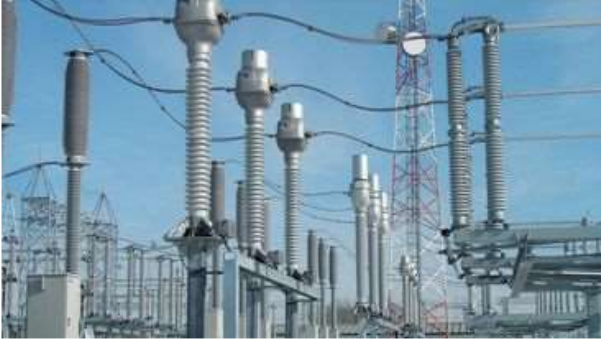
Figure 2.8: Current Transformer
