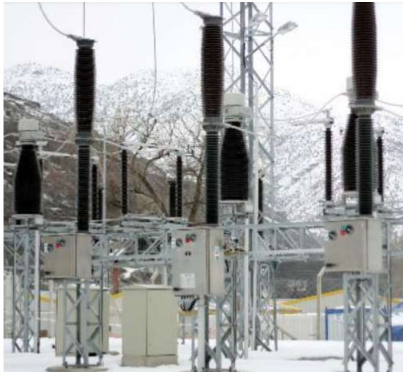
Fig2.7: Alstom High Voltage Circuit Breaker
