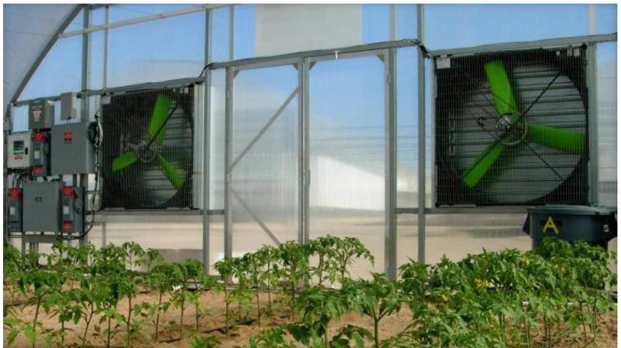
Figure 0.4 component placed in one panel
